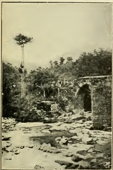
BRIDGE OVER GO-SHI RIVER.
